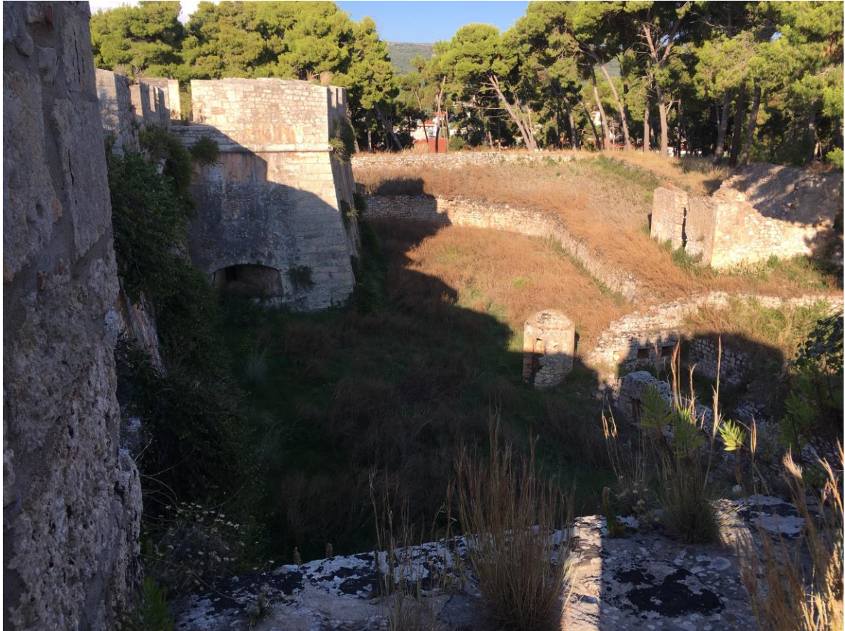
The miniature ravelin viewed from the southwest face of the citadel, showing how far into the main ditch the ravelin projects. The building directly behind the ravelin clearly has no function as a piece of fortification.
